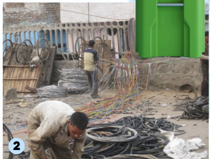
2 Workers dismantling electronics without proper protection.
